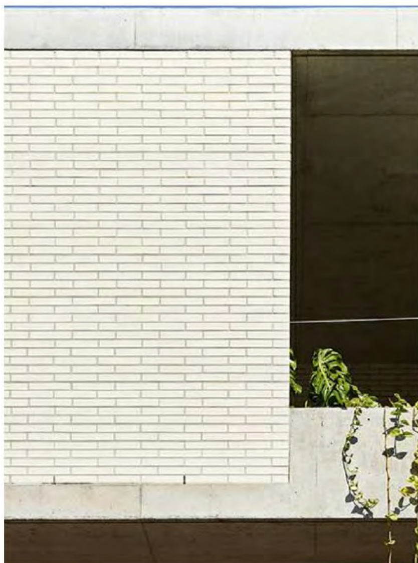
WHITE BRICK & CONCRETE
